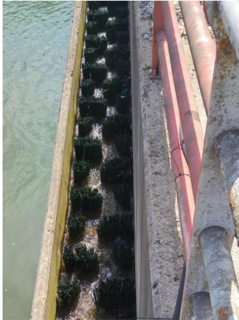
**Figure 2.** General view of the diagonal brush fish pass from downstream view at Incirli Small Hydropower Plant. The channel has a bed slope of 10% and width of 1.1 m.
