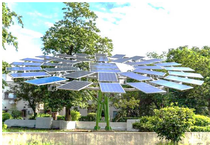
Figure 1. SPVT of 35 PV panels with a capacity of 11.55 kW (Open-source image: PIB, Govt. of India) [2].
