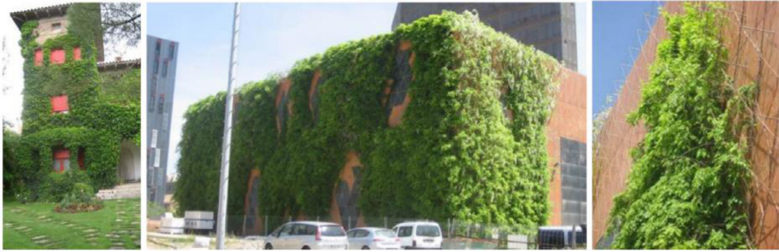
Fig. 18. Comparison of building appearances of traditional green facade (left) versus double-skin green facade [166].
