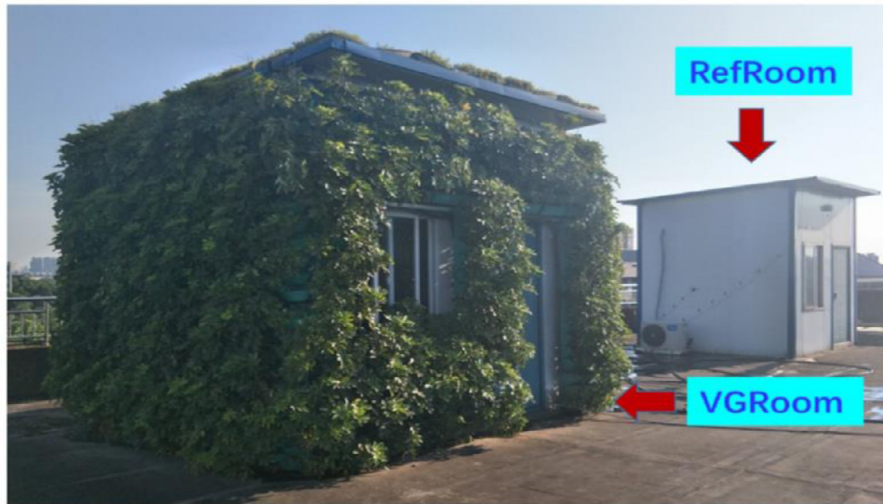
Fig. 14. VGS and green roof integrated test room and reference room [92]).
