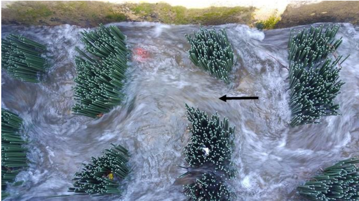
Figure 3. S flow in diagonal brush fish pass at Incirli Small Hydropower Plant. Bristle clear height is 0.37 m. Young modulus of elasticity of bristles is E = 973 MPa.
